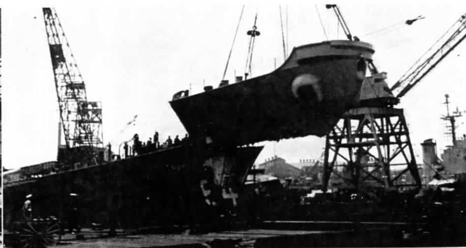
Upper undamaged portion of the Wisconsin's bow is lifted out of the way to facilitate installation of the lower section.
